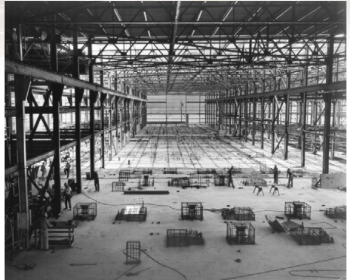
Above: One of the main process buildings during construction.
