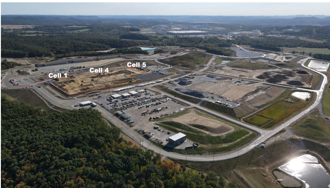
Figure 2.2. PORTS On-Site Waste Disposal Facility October 2022 (looking southwest)
